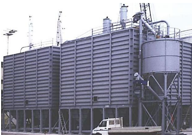
7.9-rasm. Sochiluvchan materiallar saqlaydigan bunker
