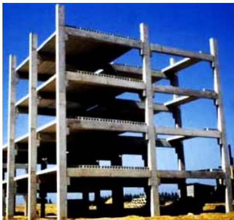
4.89-rasm. Ko`p qavatli temirbeton karkasdan iborat to`sinli sanoat binosining montaji
