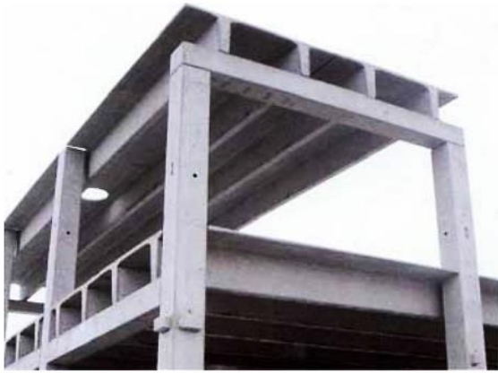
4.64-rasm. 2T turidagi to`shama panellar
