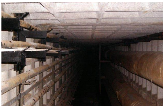
7.5-rasm. O`tish tunneli
